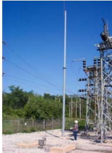
Figure 1: Traditional lightning mast protecting substation from lightning
