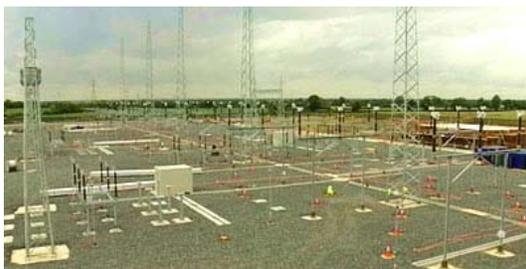
Figure 2: Low profile substation (Source: POWERTEAM Electrical Services)
