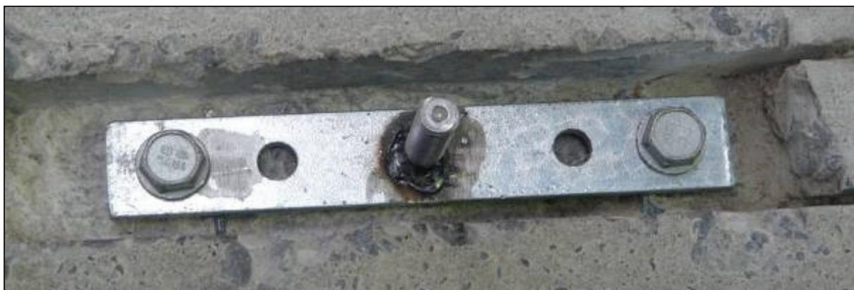
**Photo 2: Earthing bracket for Hollow spun pole, prior to grouting, showing connection to two binding wires.**
