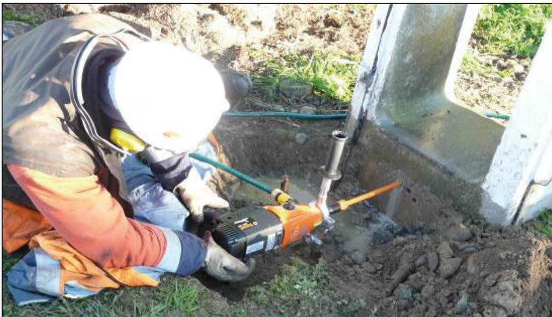
*Photo 4: Diamond drilling a Vierendeel pole.*
