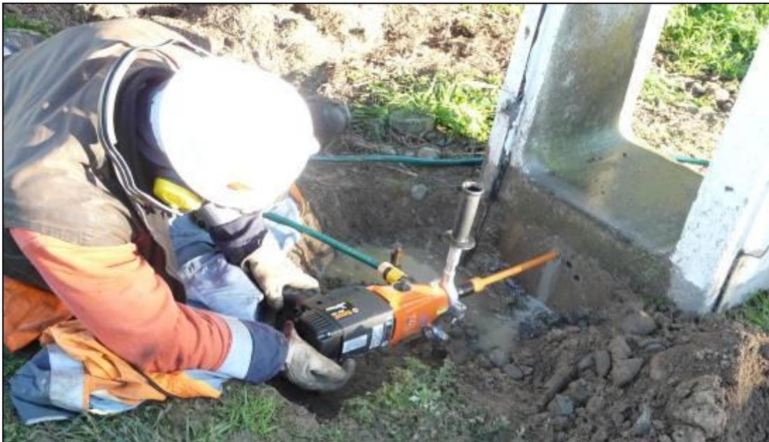
*Figure 5: Diamond drilling a Vierendeel pole.*
