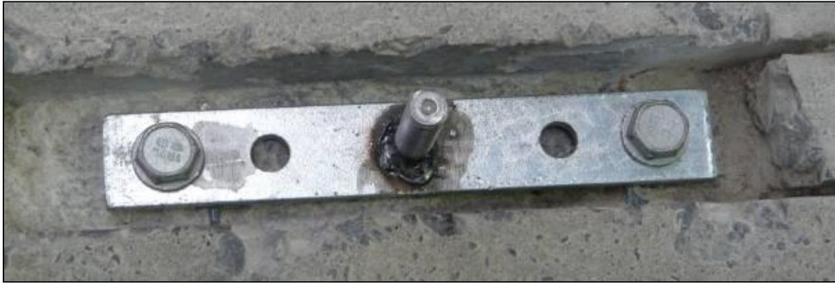
**Figure 8: Design 1A Bonding Bracket for Hollow Spun Poles.**
