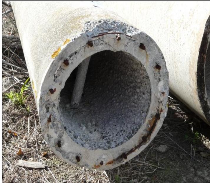
*Figure 7: Hollow spun pole top cross-section with cap removed showing ends of vertical prestressing strands, and portions of spiral binding wire*
