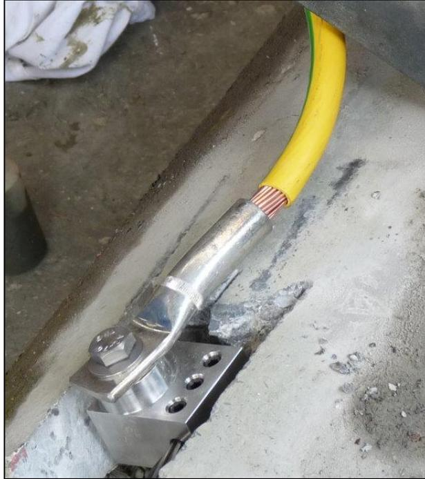
**This paper rounds up three years of investigation, design, development, testing and field trialing of methods of earth bonding the reinforcing cages of older Vierendeel and hollow spun concrete poles which were manufactured without integral earthing systems.**
