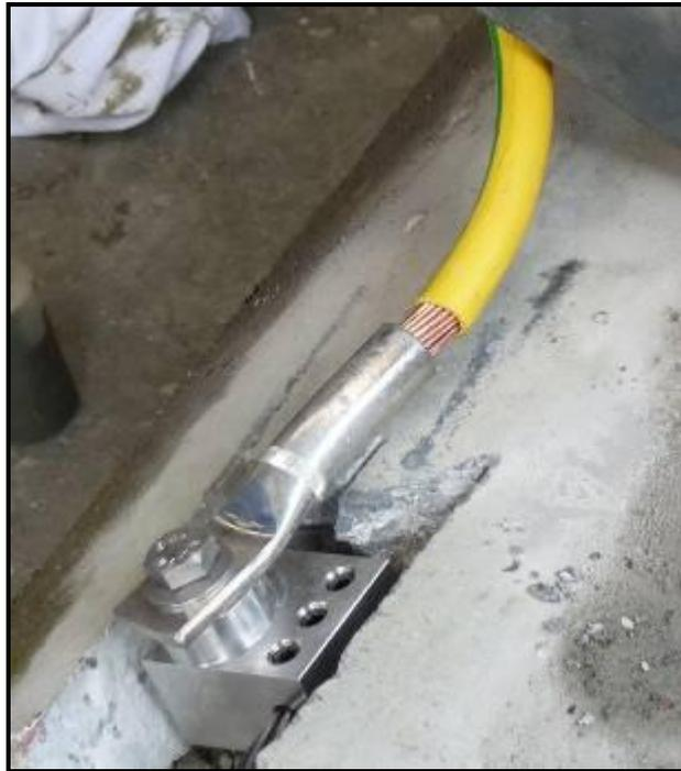
*Figure 10: Hollow Spun Pole top bonding connector (Prior to mortaring into pole wall).*
