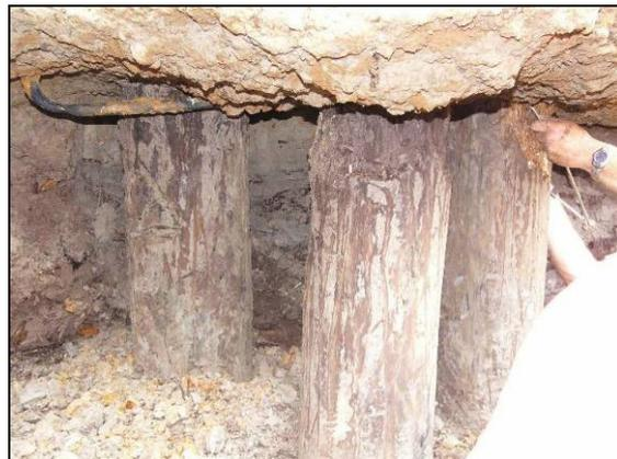
**Photo 2: Three timber piles under the concrete**
