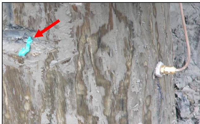
**Photo 7: Internal preservative oozing out a grub hole.**
