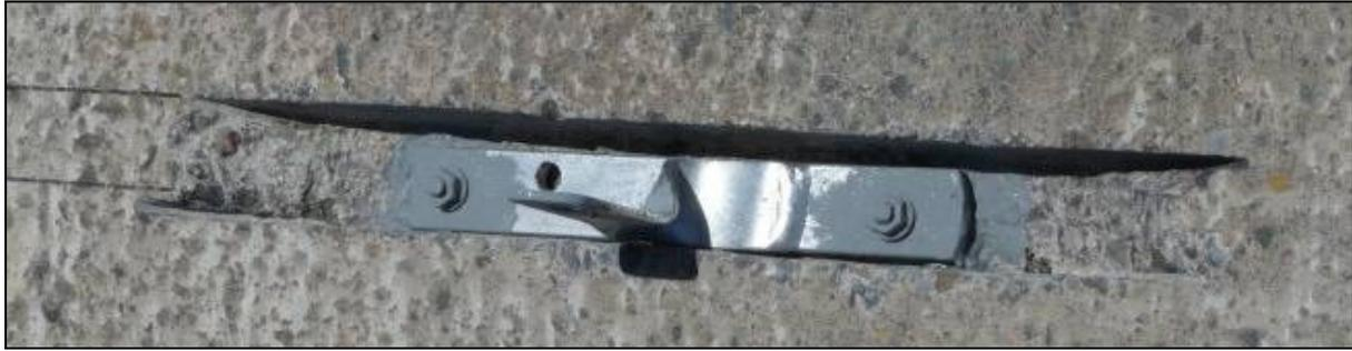
**Photo 8: An early prototype bracket installed on a hollow spun pole, prior to reinstatement with mortar.**
