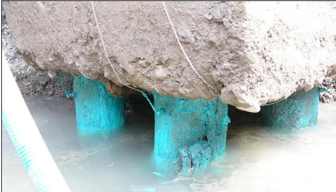
**Photo 5: Injection lines installed and external pile surface coated with preservative.**
